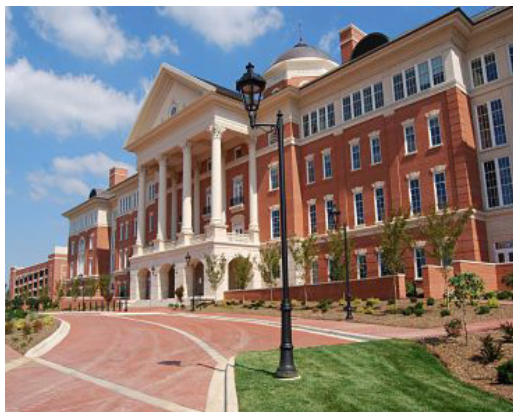
DAVID H. MURDOCK CORE LABORATORY BUILDING
